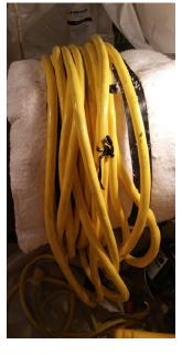
Preheat - keep cable off of pipe with fire blanket or wood stakes
