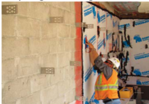
Applying a single ply membrane wrap to concrete masonry unit (cmu)
