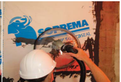
Penetrations and membrane seams/joints are tested
