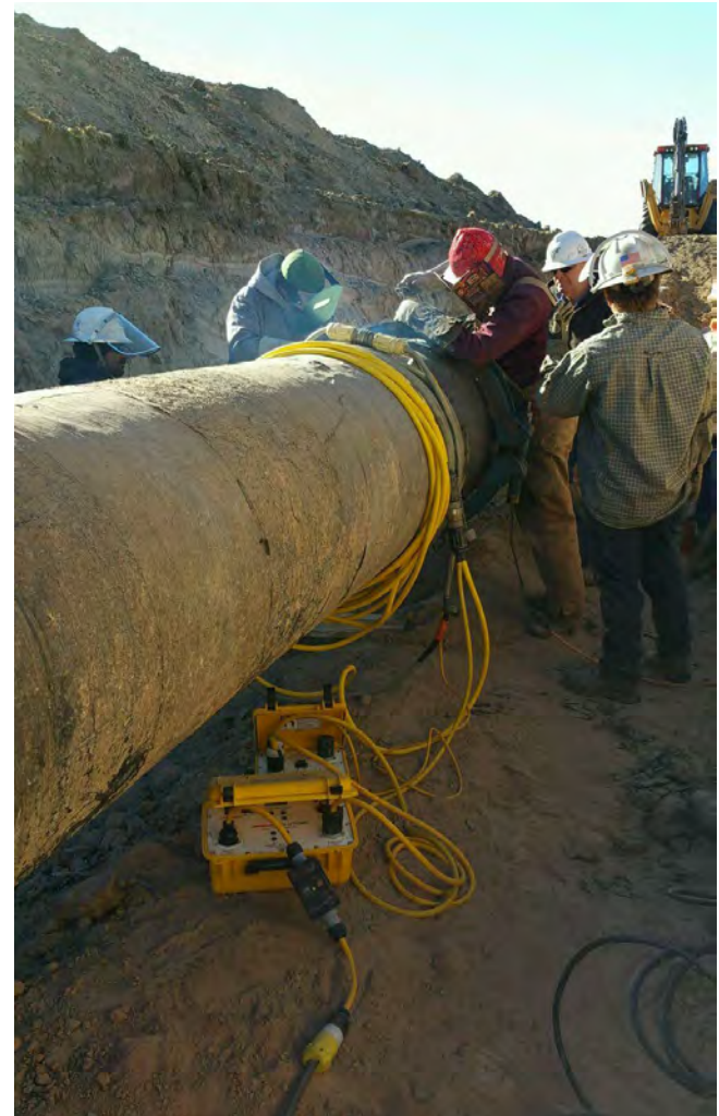
Using the DEMAG to make the root pass
