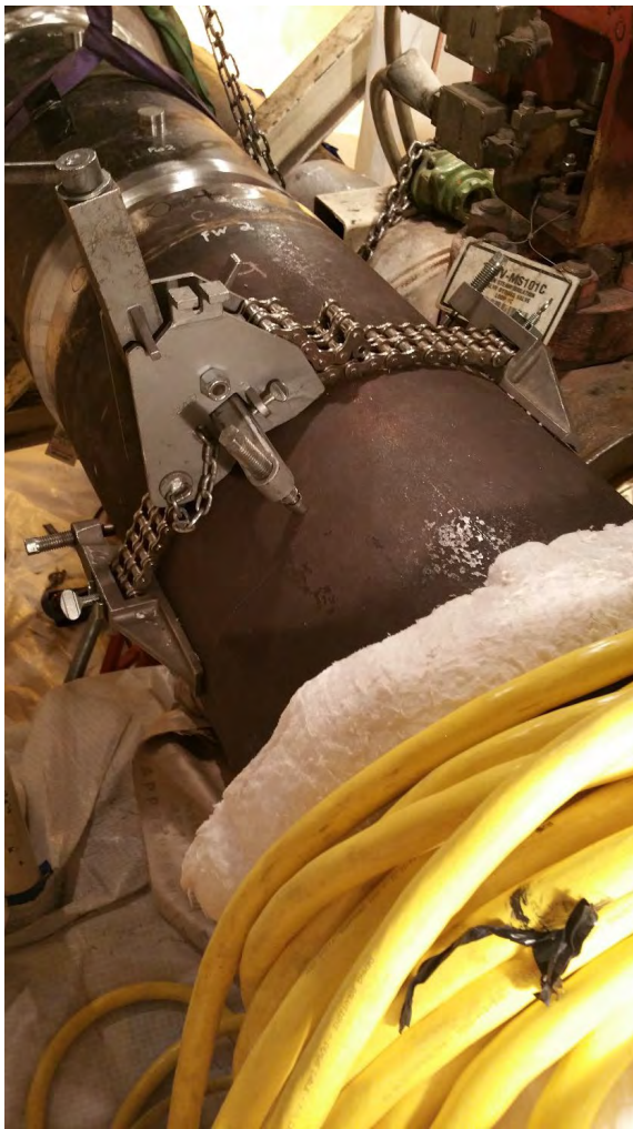
Demagnetizing cable wrapped on a fire blanket for protection from pre-heat
