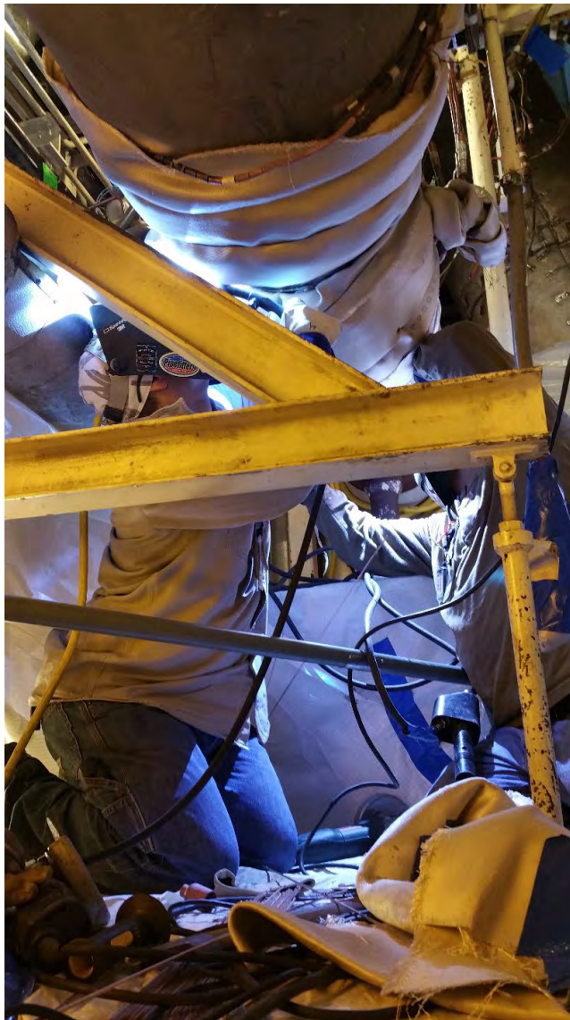
Cable wrapped on fire blanket
