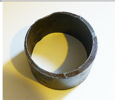
Figure 17 Severe Eroded Pipe Wall
