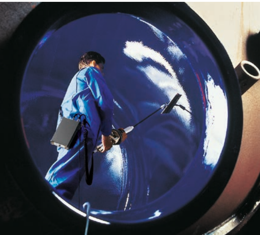
Pore testing of the enamel coating of a boiler, using the POROSCOPE®
