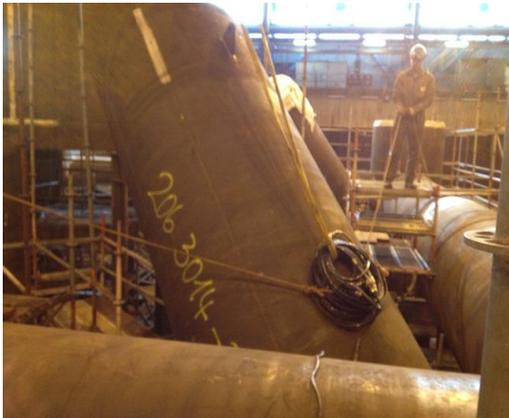
Demagnetization of construction pipes
