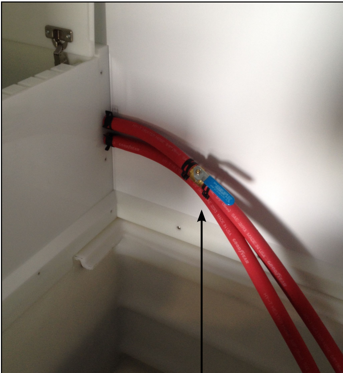
Chill chaser valve shown in the open position
