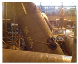
Demagnetization of construction pipes
