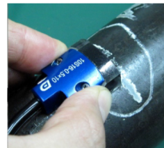
Small Diameter Pipe Welds
