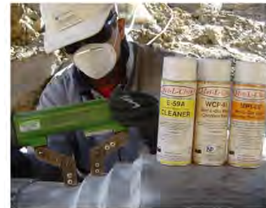
Pipe line inspection using MPI-80
